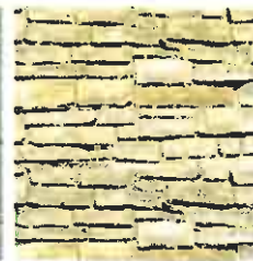
Gateway Monument Wall Stone Veneer
