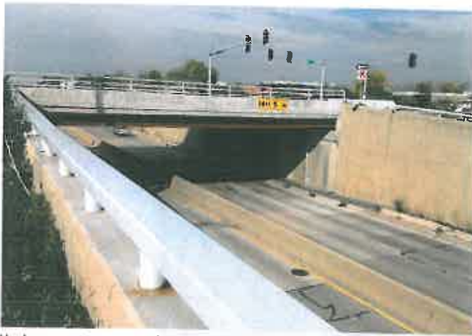
Underpass structure and retaining walls are an opportunity for community identity signage
