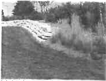
Embankment Limestone Retaining Wall Precedent
