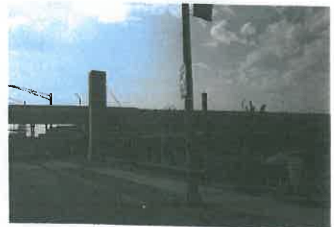
Palatine Road bridge is an opportunity for landscape and signage enhancements
