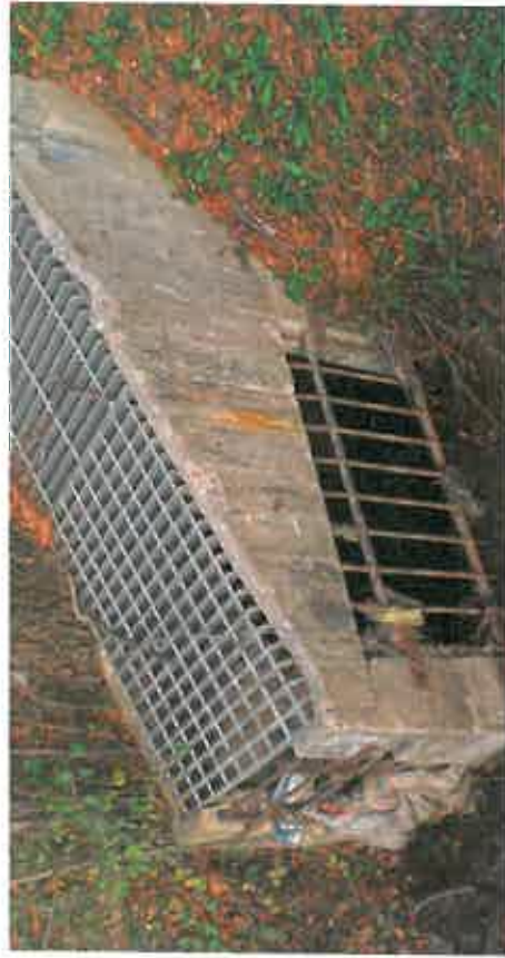
Figure 2.16: Stormwater intake
