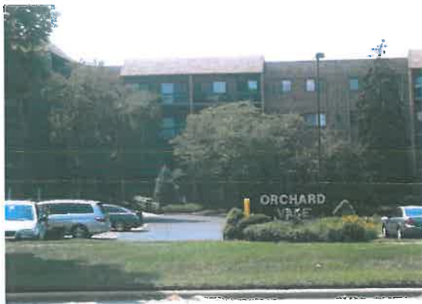
4-Story Orchard Vale condos on Elmhurst Road – 1.59 ESE
