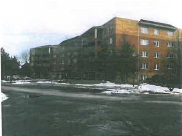
5-Story Apt Building – 1.25 Miles S of site along Rand Road
