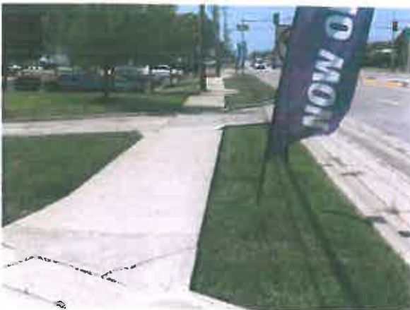
Sidewalk Improvement: View looking N
