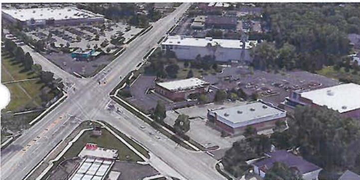
Aerial View from Northwest
