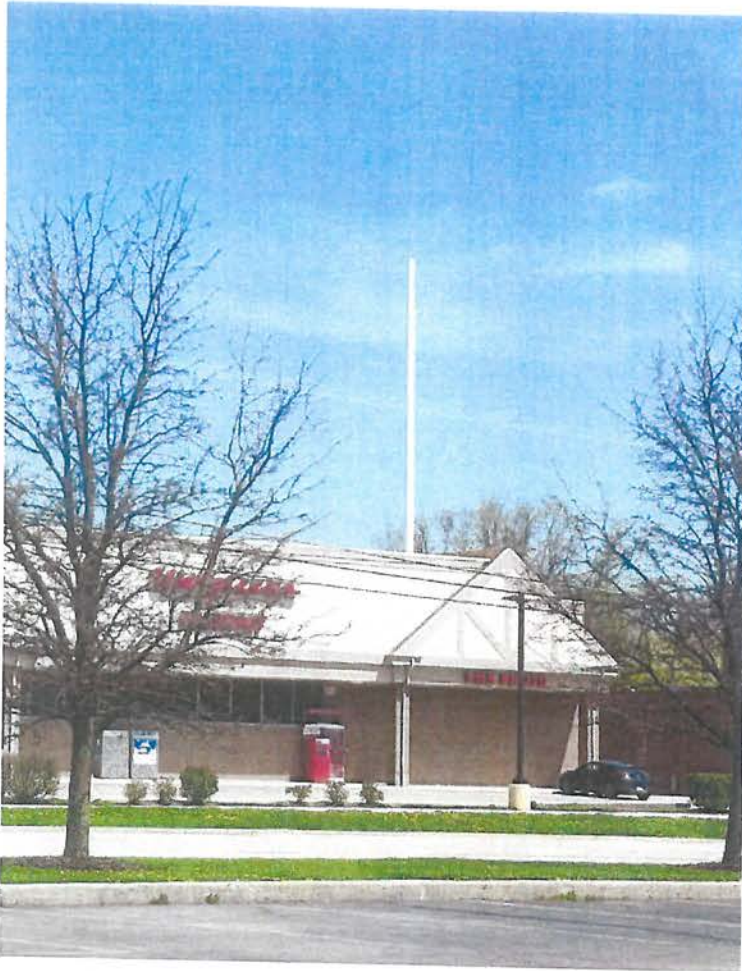
Current "Concealed Antenna"
