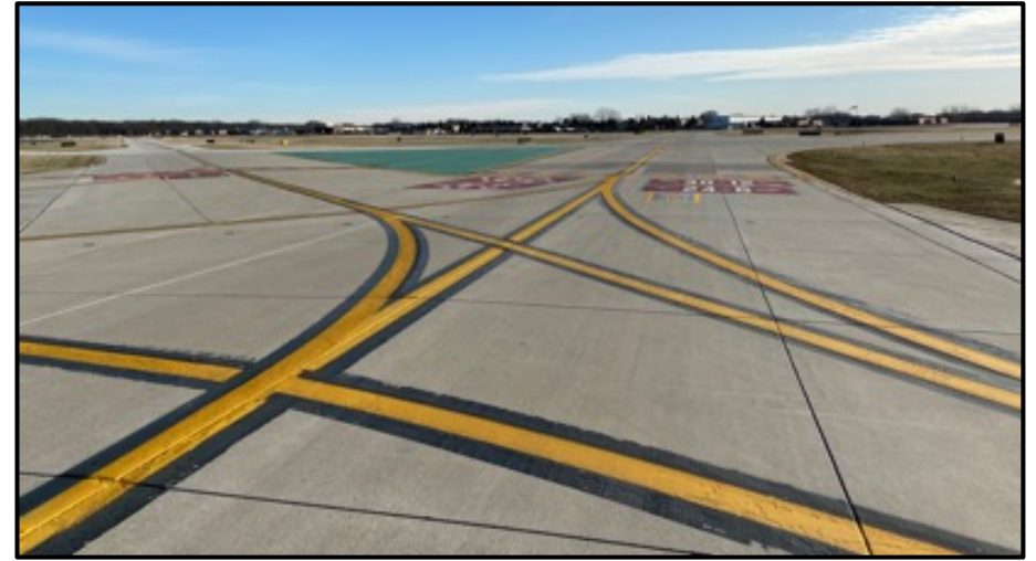
Hot Spot #1 ground view
