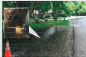
STONEGATE DRAIN TILE REPAIR
